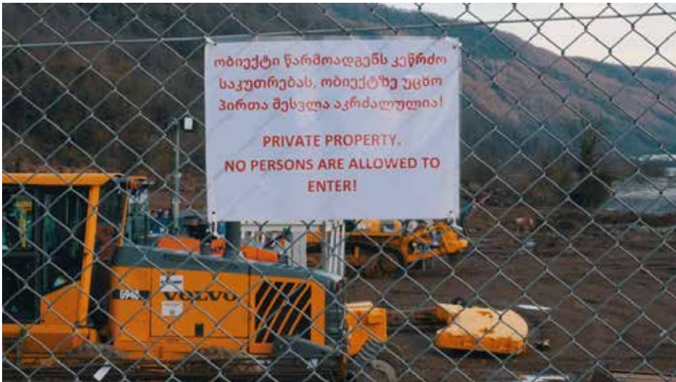
Construction Site of the Namakhvani HPP (Photo: Social Justice Center)
